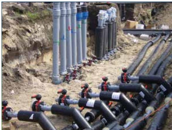
Flexible, pre-insulated pipe system for geothermal applications such as ground source heat pumps.
